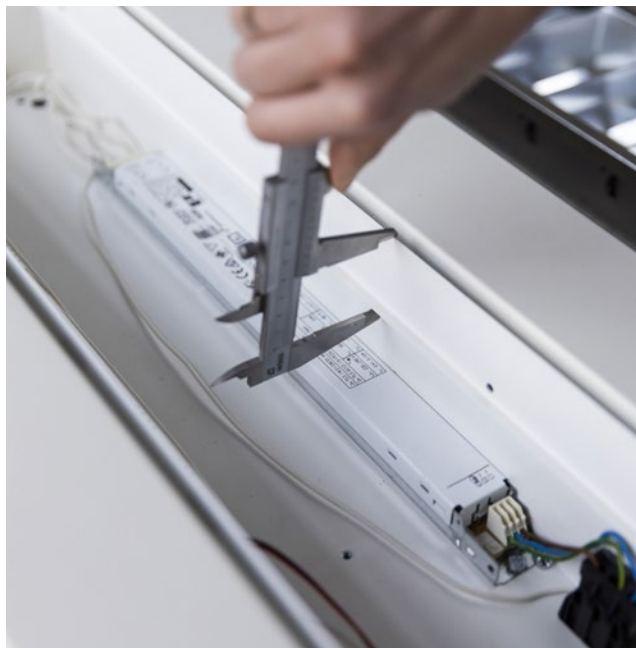
Step 2: Measurement of the existing casing to design optimal fixing system
